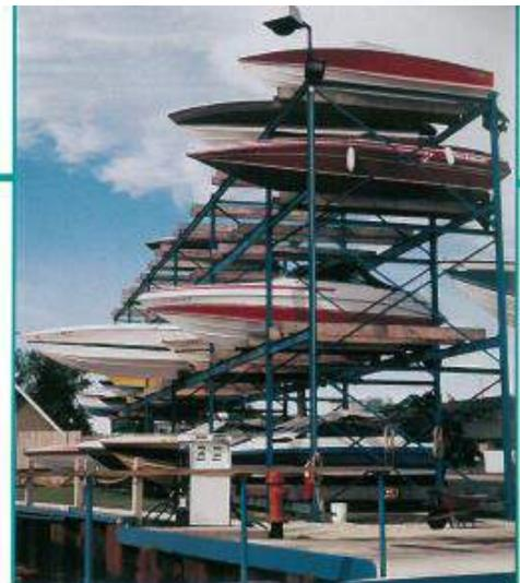
All of our boat racks are manufactured from structural steel and designed in accordance with latest editions of the American Institute of Steel Construction (AISC), Rack Manufacturers' Institute (RMI), and Metal Building Manufacturers' Association (MBMA).
